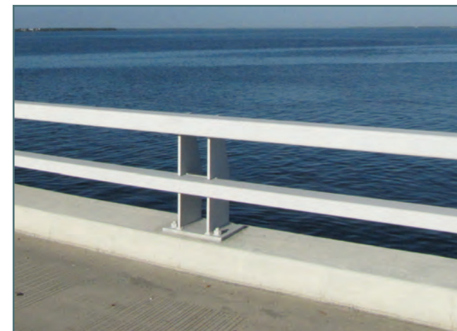
Example of Wyoming Railing
