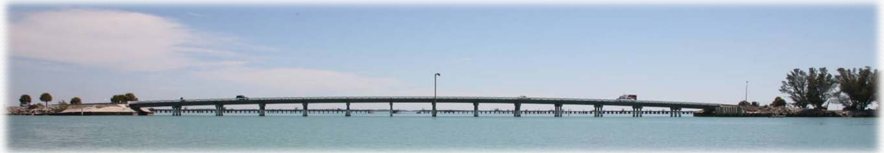
Existing vertical clearance = 15 feet
